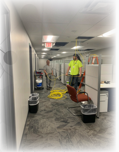
Fiber installation in Springfield
