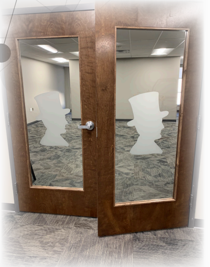
Entry doors at 524 S. 2nd, Springfield
